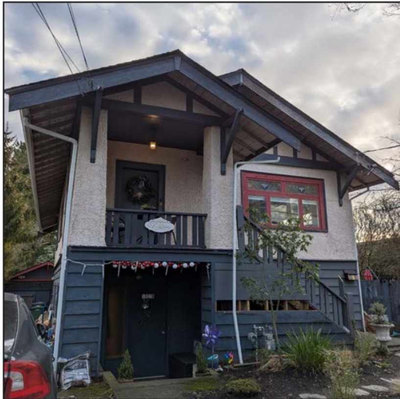
Fig. S1: Front view of 1527 Redfern Street, 2024. (Source: Cummer)
