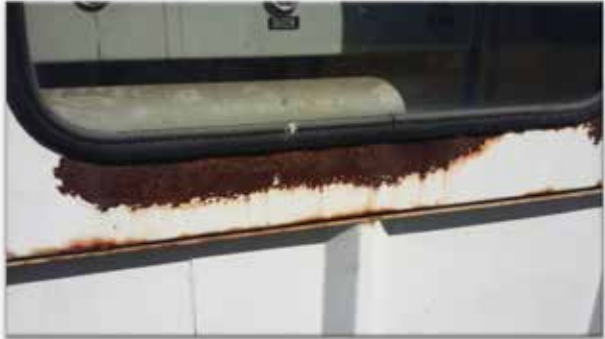
Enclosure corrosion
