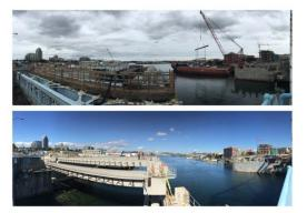
installed large concrete sections that now form the road approaches leading up to where the new steel structure will sit.
