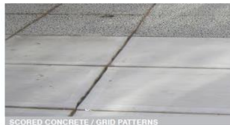
SCORED CONCRETE / GRID PATTERNS
