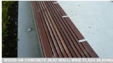
WOOD ON CONCRETE SEAT WALL: WIDE PLAZA SEATING
