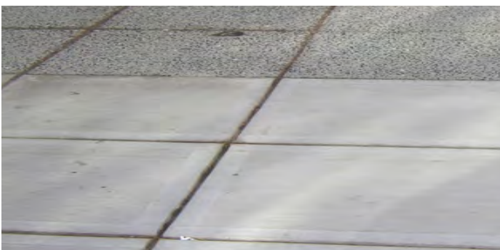
SCORED CONCRETE / GRID PATTERNS
