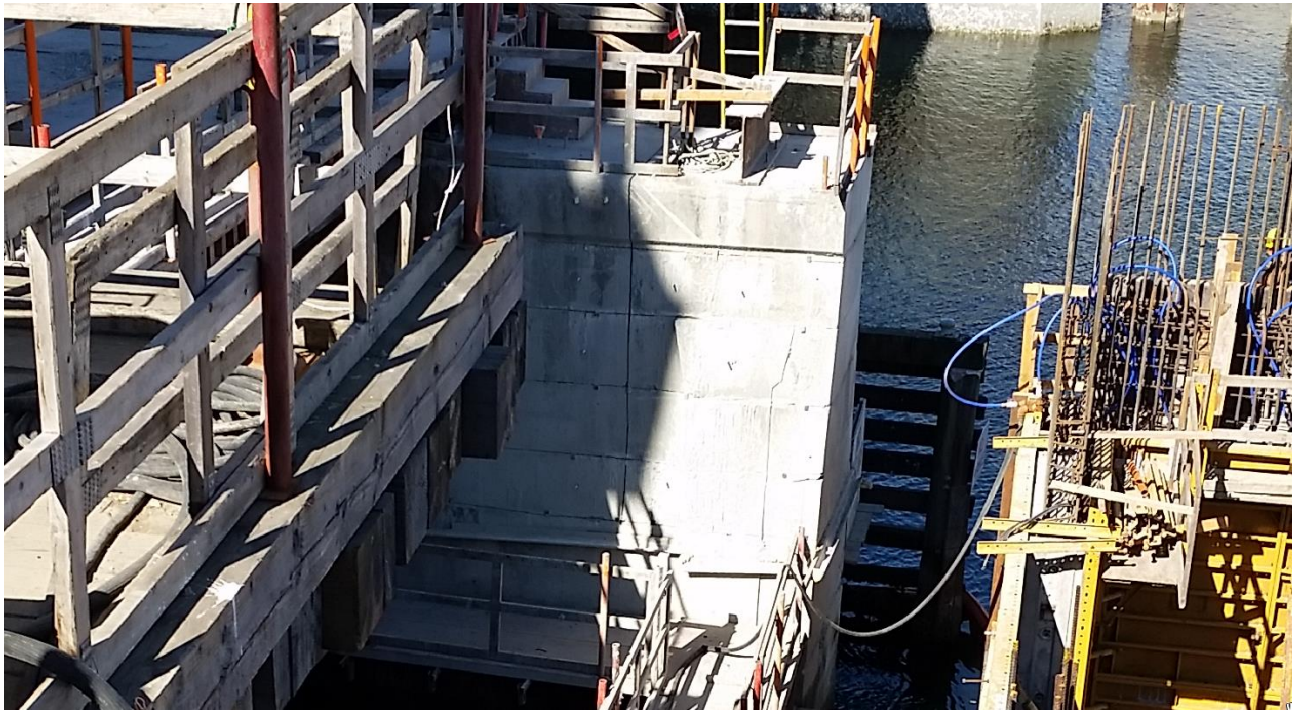
East side Rail Span Pier can be seen cut into blocks in place ready for removal by crane.
