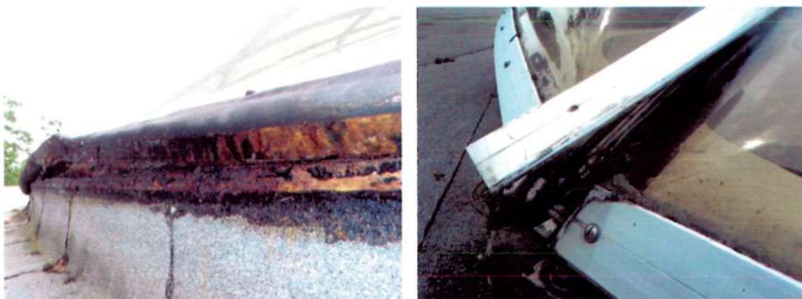
Figure 3: Photos showing poor condition of existing domes
