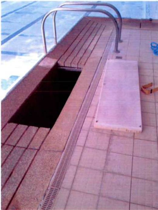
Figure 8: The only existing rim flow access
