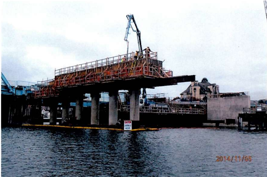
West side rest pier during concrete pour November 5, 2014
