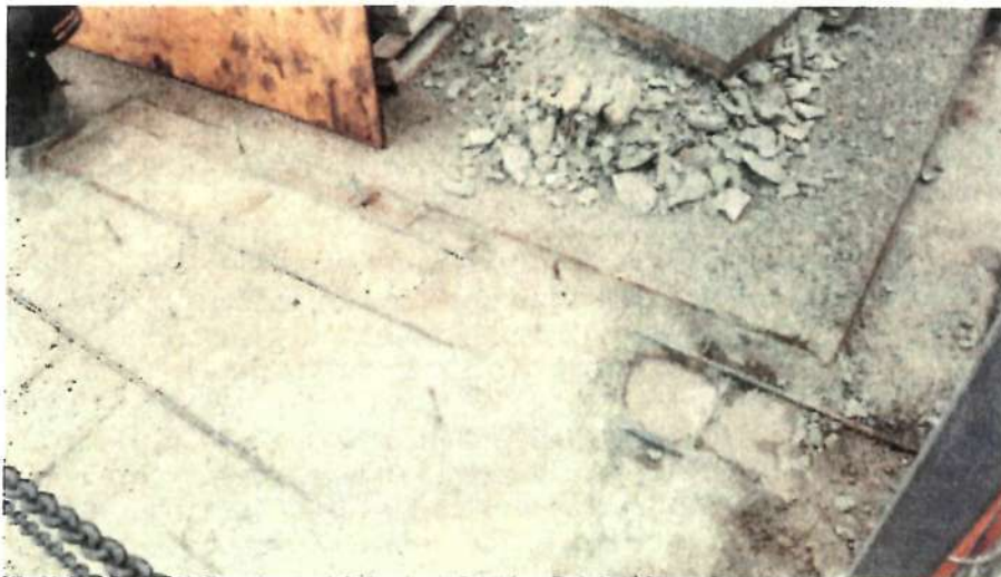
Image 1: Top Reinforcing at Existing Slab. May 4, 2017
