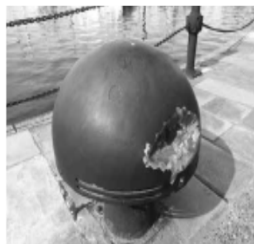
Damaged lights
