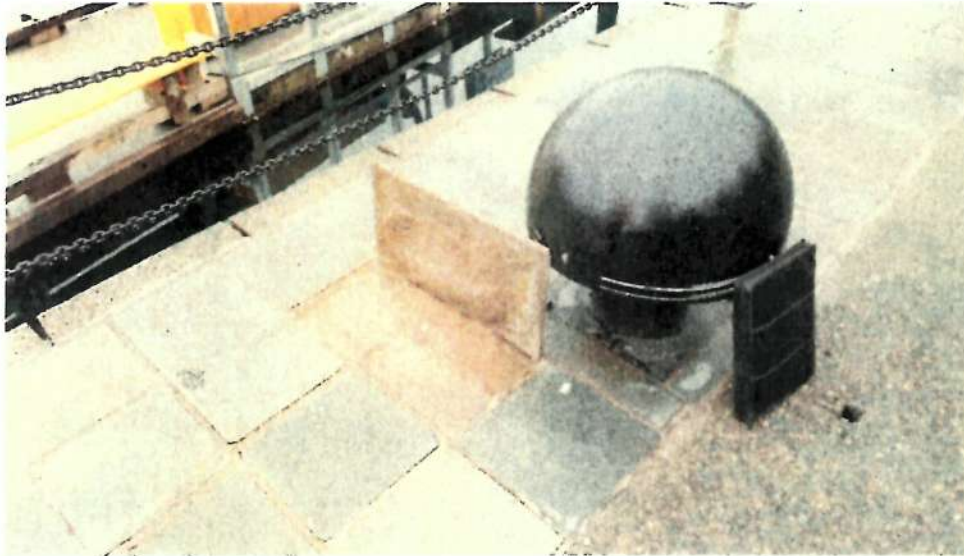
Image 3: Un-bonded 2014 Pavers and Existing "Mushroom" Light
