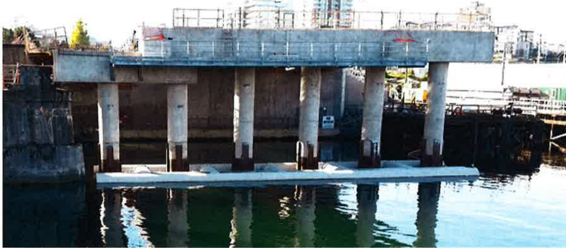
Floating rest pier can be seen at water level. This protection device rises and falls with the tide.
