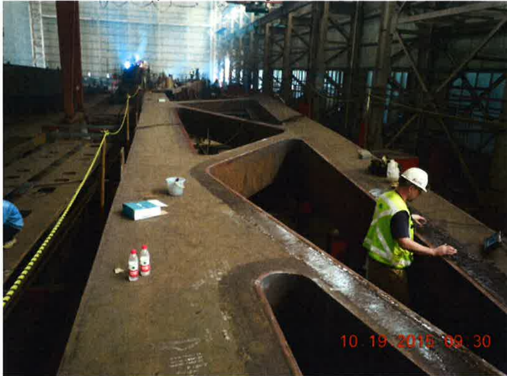
Photo 2 – Orthotropic steel deck end floor beam assembly and welding
