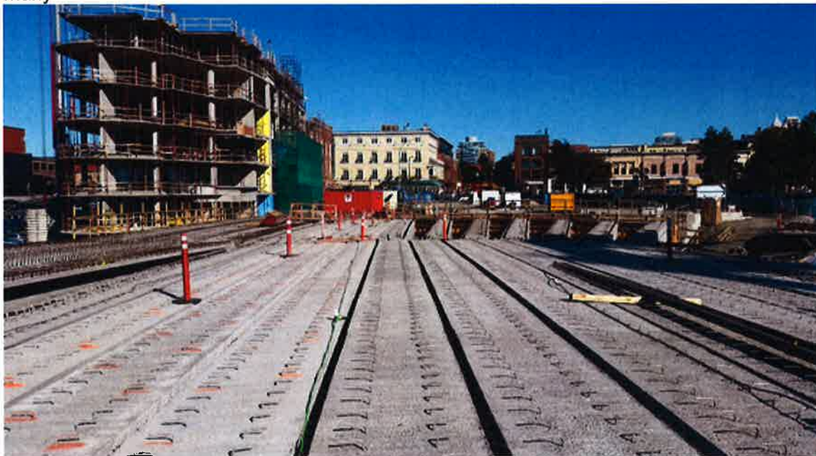
View from the edge of the bascule pier up Pandora. Girders seen will form the deck of the new bridge.
