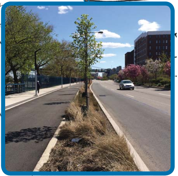
Install an eco- median along one side of the cycle track. This one is in Philadelphia.
