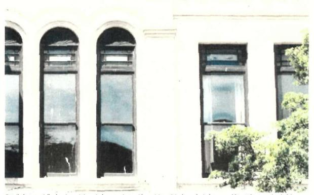
Detail photo partially showing existing window openings, with surviving original wood window assemblies at the upper level of the historic street facade.
