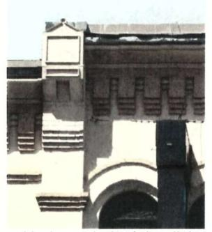
Detail photo showing typical condition of architectural brickwork detailing and metalwork along parapet level.
