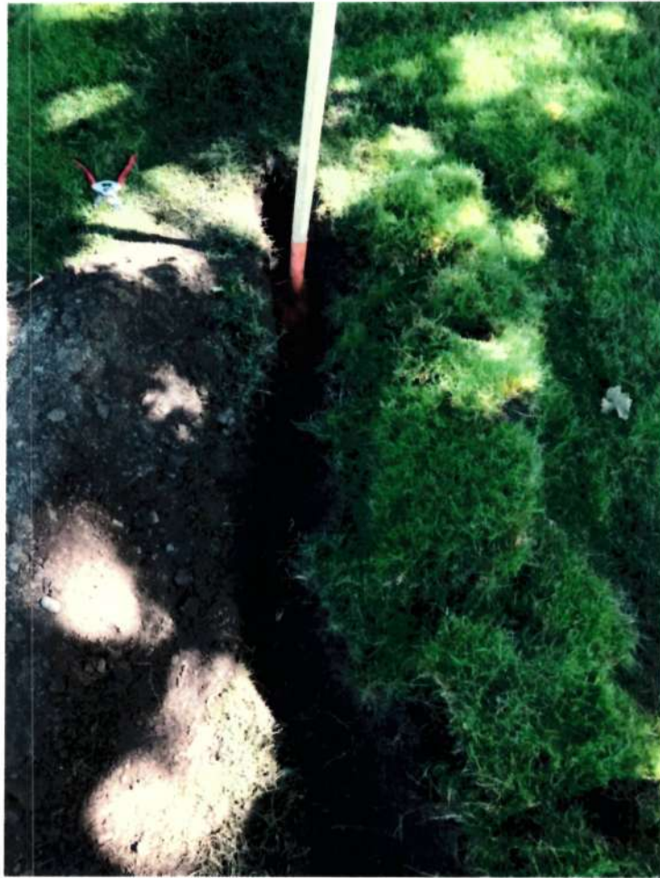
Image 2. Two 2cm diameter roots, fifteen 1cm roots, and a high density of fibrous roots were encountered along the entirety of the trench (approximately 4m).
