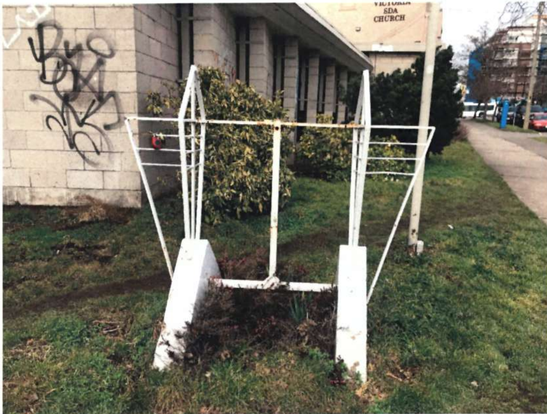
Identification sign with concrete base and an iron flat-bar structure
