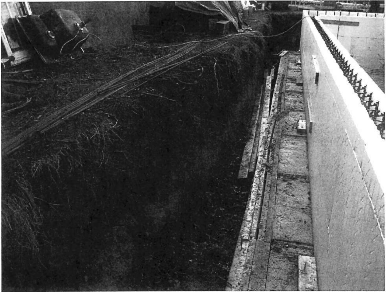
Picture 1: View of edge of excavation showing no large roots exposed (picture supplied by client).
