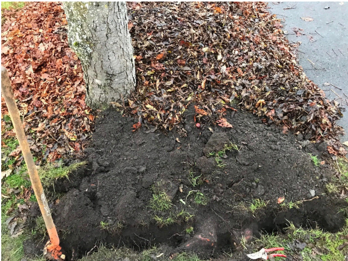
Photo 3: Exploratory excavation adjacent to NT #3.
