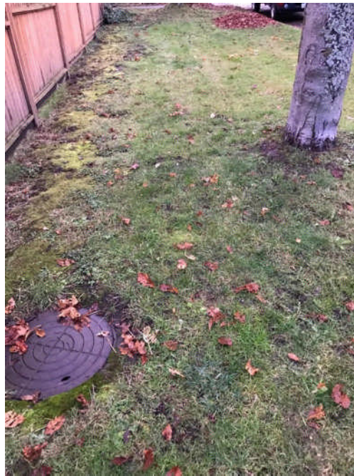
Photo #7: A water meter is located east of Red Horse Chestnut NT #2. If this water meter opening can be raised to meet the grade of the sidewalk, we are not aware of a reason why the sidewalk could not be raised above the root system.
