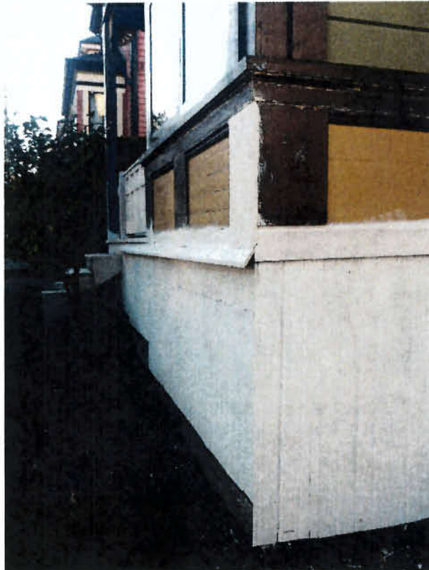
Vertical skirting boards at foundation level
