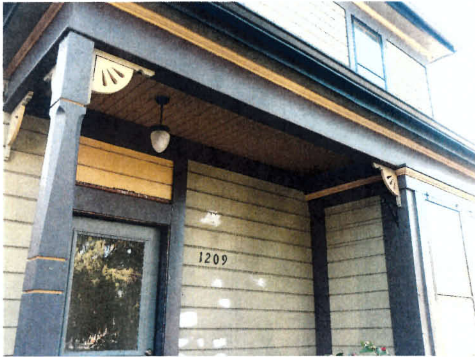
Scroll cut brackets and chamfered porch post
