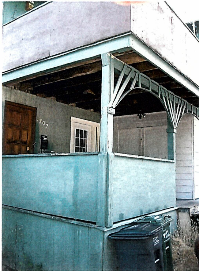
View of fan brackets on rear addition
