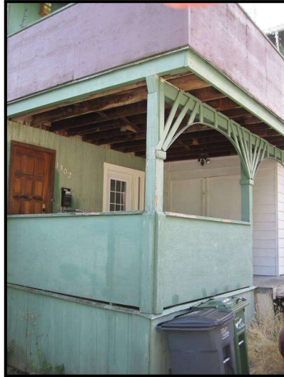
Fan Brackets on 1976 Addition
