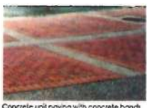
Concrete unit paving with concrete bands
