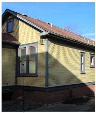
2x 1-over-1 double-hung wood sash w/ horns Treatment: Rehabilitation, as necessary
