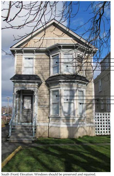
1-over-1 double hung wood sash w/ horns 1-over-1 double hung wood sash w/ horns
