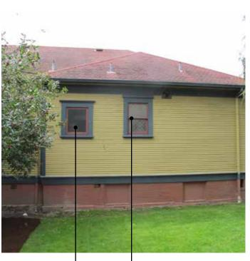
**1x 1-over-1 double-hung wood sash** Treatment: Rehabilitation, as necessary
