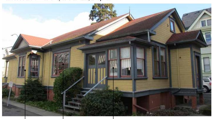
**2x 1-over-1 double-hung wood sash** Treatment: Rehabilitation, as necessary
