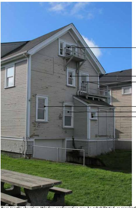
2x 1-over-1 double hung wood sash w/ horns 1-over-1 single hung wood sash Casement (fire egress)
