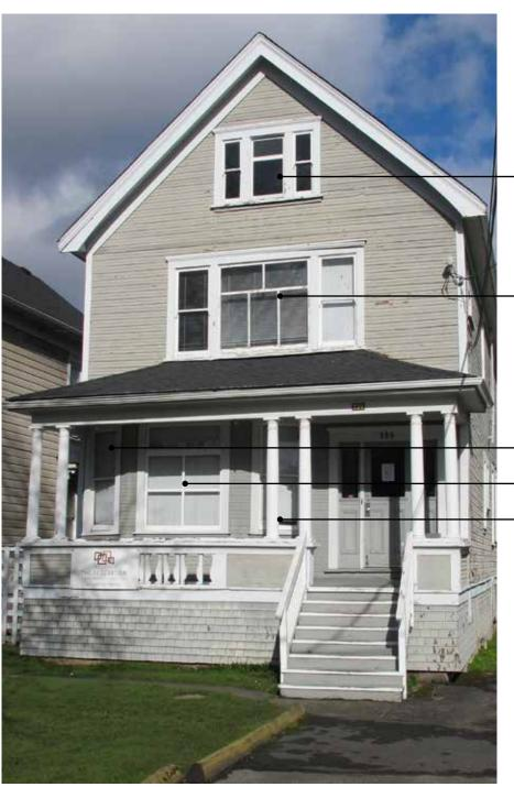
2x 1-over-1 double hung wood sash w/ horns 1-over-1 single hung wood sash
