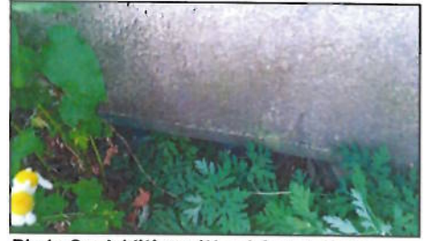
Photo 3 - Addition without foundations
