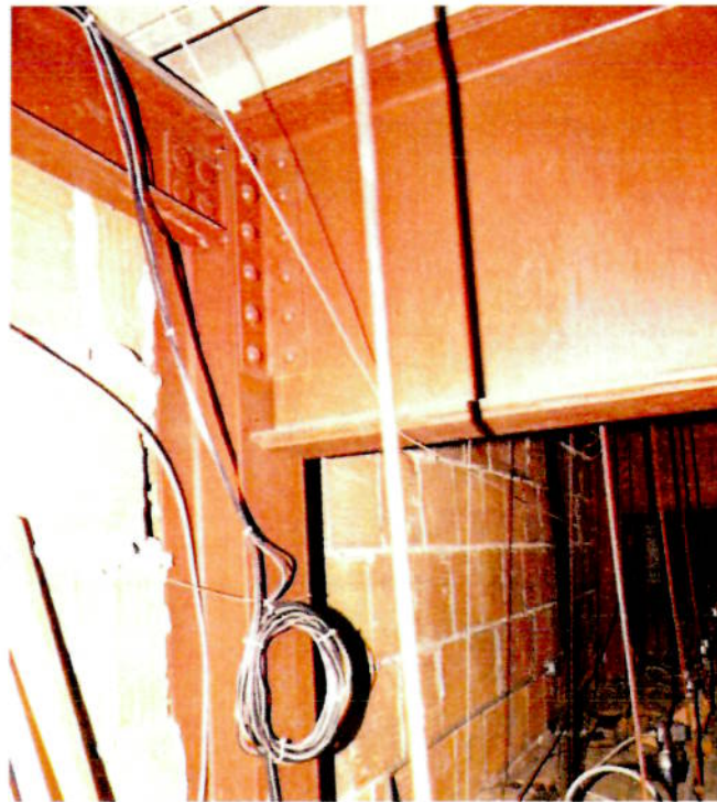
Steel structural column, girder, and beam between the roof and finished ceiling
