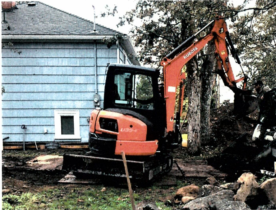
Image 14: Rubber tracked mini excavator on plywood sheets.
