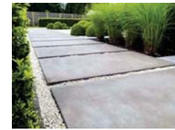
CIP Concrete Path with permeable gravel edging
