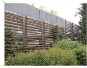
1 Example of Metal and Wood Slat Screen
