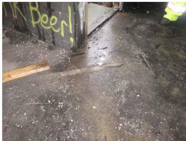
No. 10 – Slab cracking
