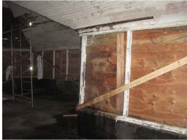
No. 6 – Wall bracing, racking and outward thrust
