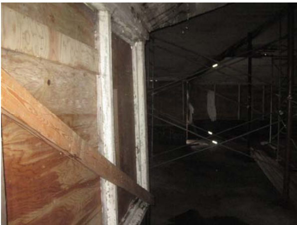
No. 7 – Wall bracing, racking and outward thrust
