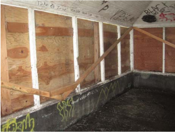
No. 5 – Interior wall bracing
