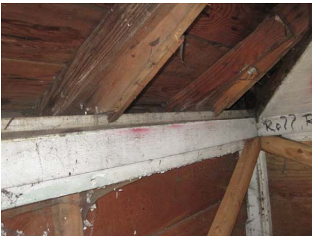
No. 3 – Header over window and rafter tails
