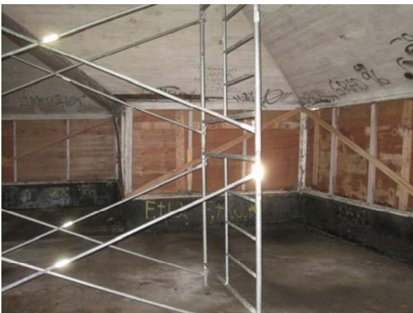
No. 9 – Wall bracing, racking and outward thrust
