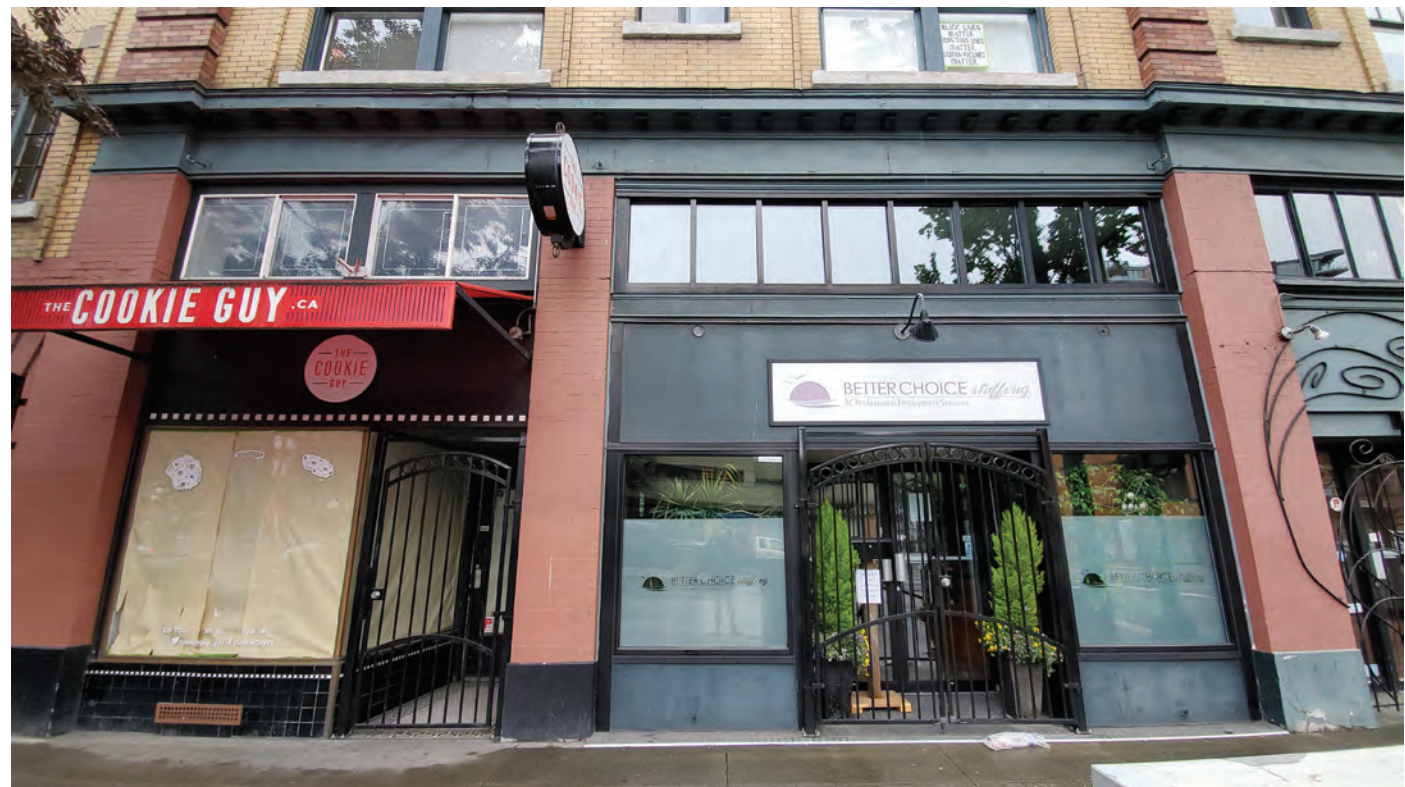
Figure 26: Detail photo showing existing typical condition of storefronts along Blanshard Street. Note ribbon of transom windows above "The Cookie Guy" does not reflect original configuration as shown above "Better Choice Staffing".
