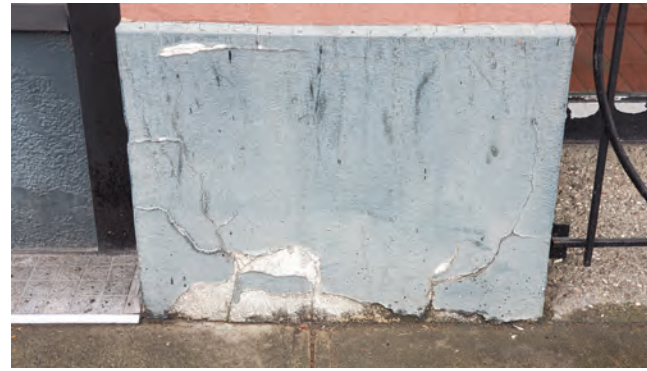
Figure 23: Detail photo showing existing typical deteriorated condition of column bases.
