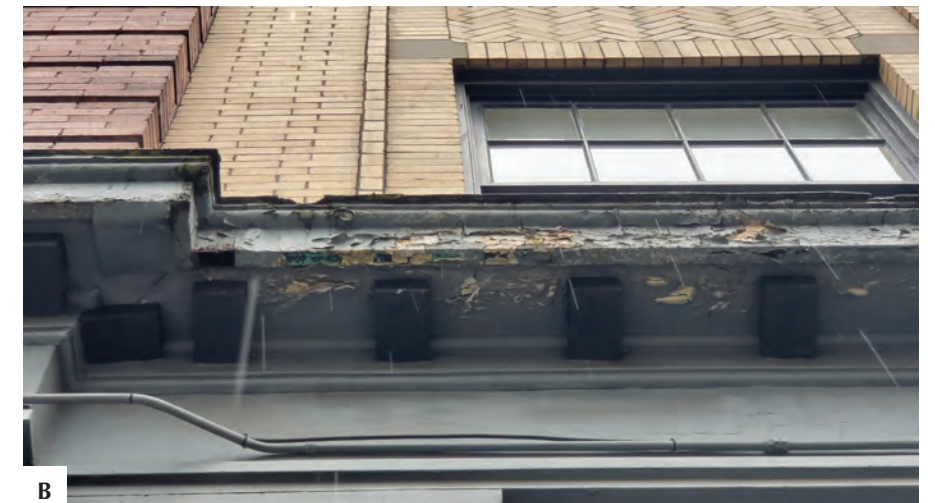
Figure 30: Detail photo showing typical deterioration of architectural metal cornice. Note discolouration and biological growth; paint failure; and, corrosion of metal elements.
