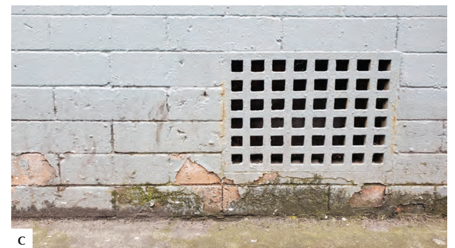
Figure 31: Detail photos showing unsympathetic paint finish over brick masonry units. Note discolouration and biological growth; further investigation is required to determine if face brick are spalling underneath.
