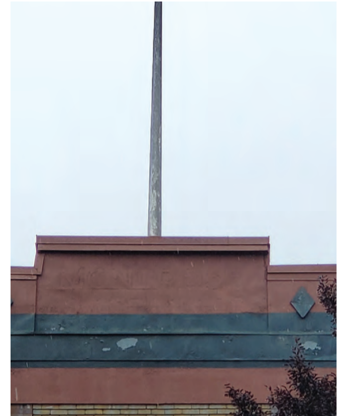
Figure 25: Detail photo showing existing typical deteriorated condition of pediment above the central bay of the historic front facade along Blanshard Street. Note existing flagpole partially shown in the background.
