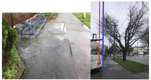
**Picture #1** (left) showing the cracks likely caused by roots of Horse Chestnut #2. All roots within private property will be removed due to the underground parkade excavation to the property line (the edge of the concrete sidewalk at the top and bottom of the photo).
