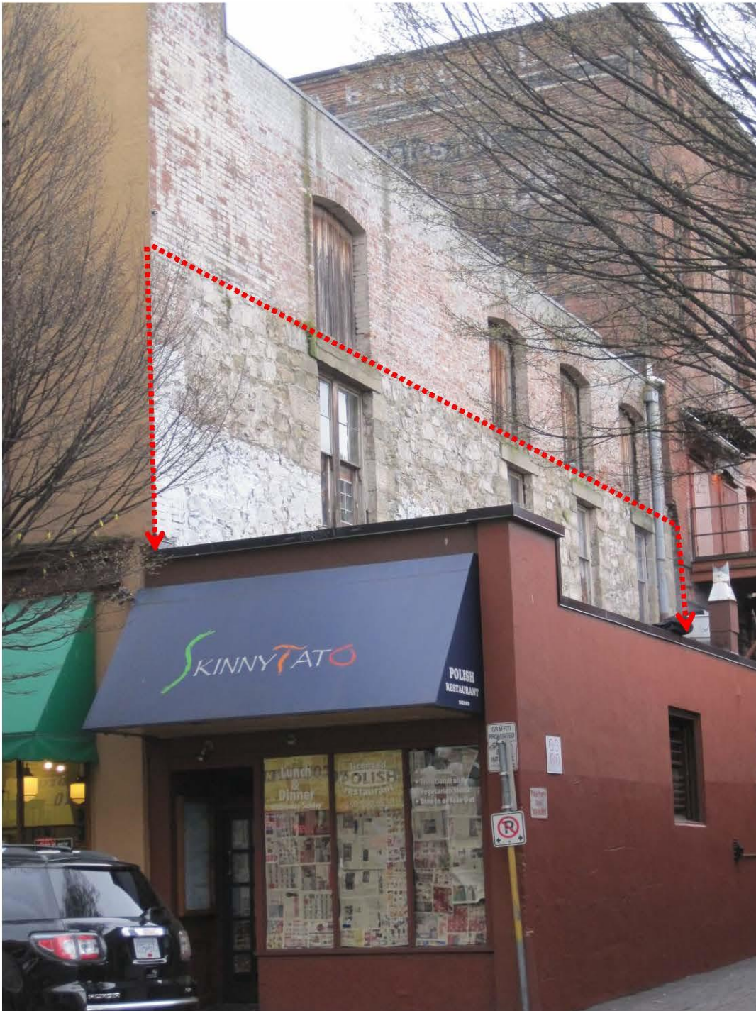
Photograph of Visible Portions of the Rubble Wall
