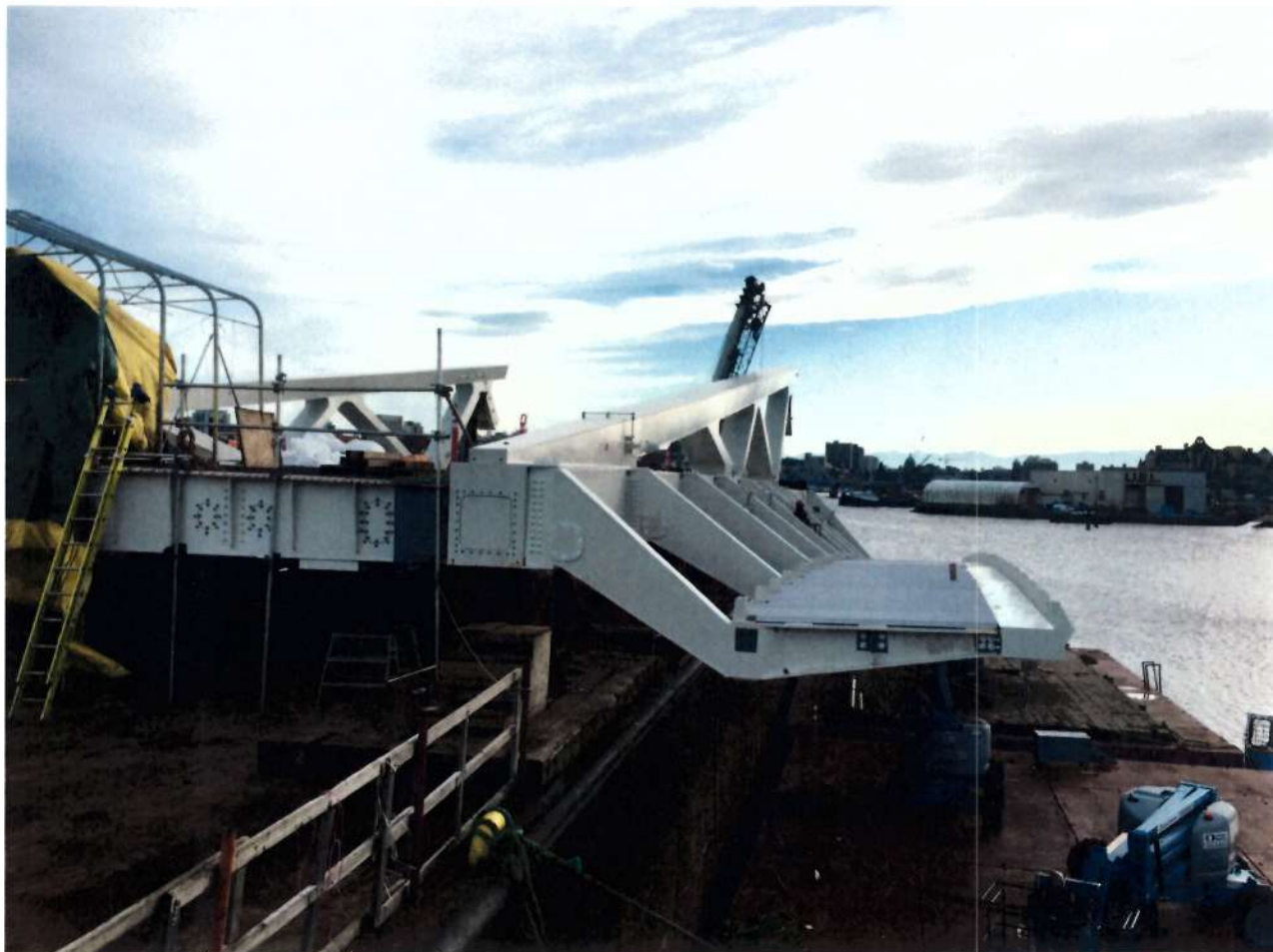
Figure 4 – Current Status of the Bascule Leaf and associated outriggers
