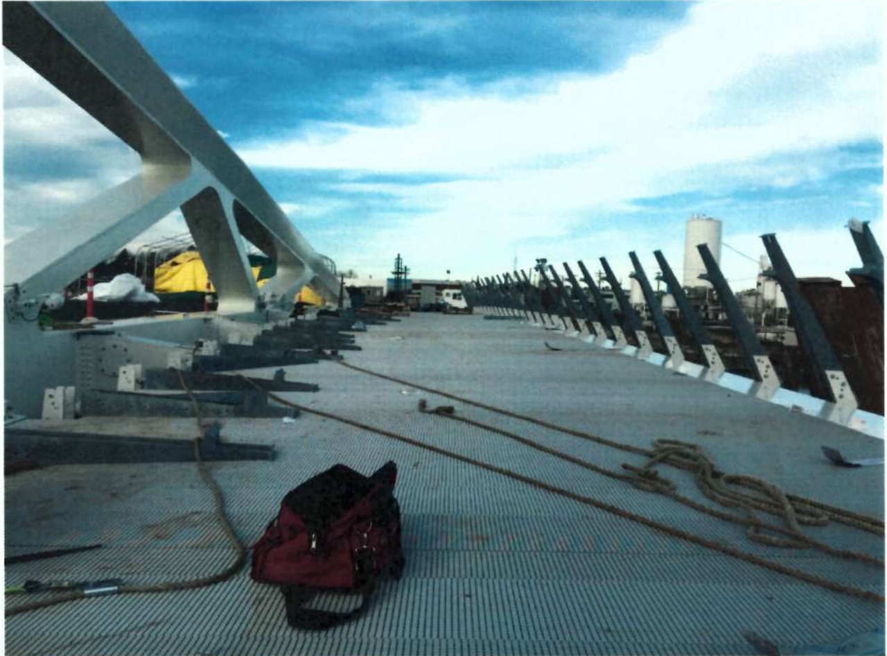
Figure 5 – MUD Deck Surface for Bascule span
