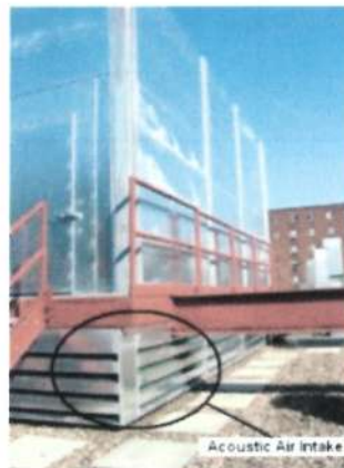
Acoustic Louvers on Rooftop Chiller Enclosure
