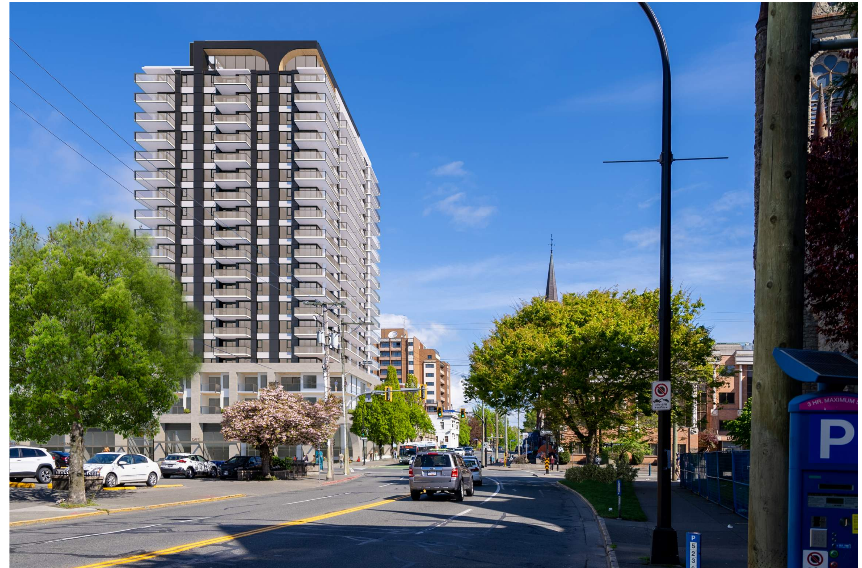
LOOKING NORTH ON QUADRA ST.
