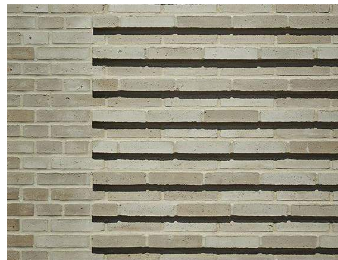
HORIZONTAL BRICK REVEAL DETAILING
