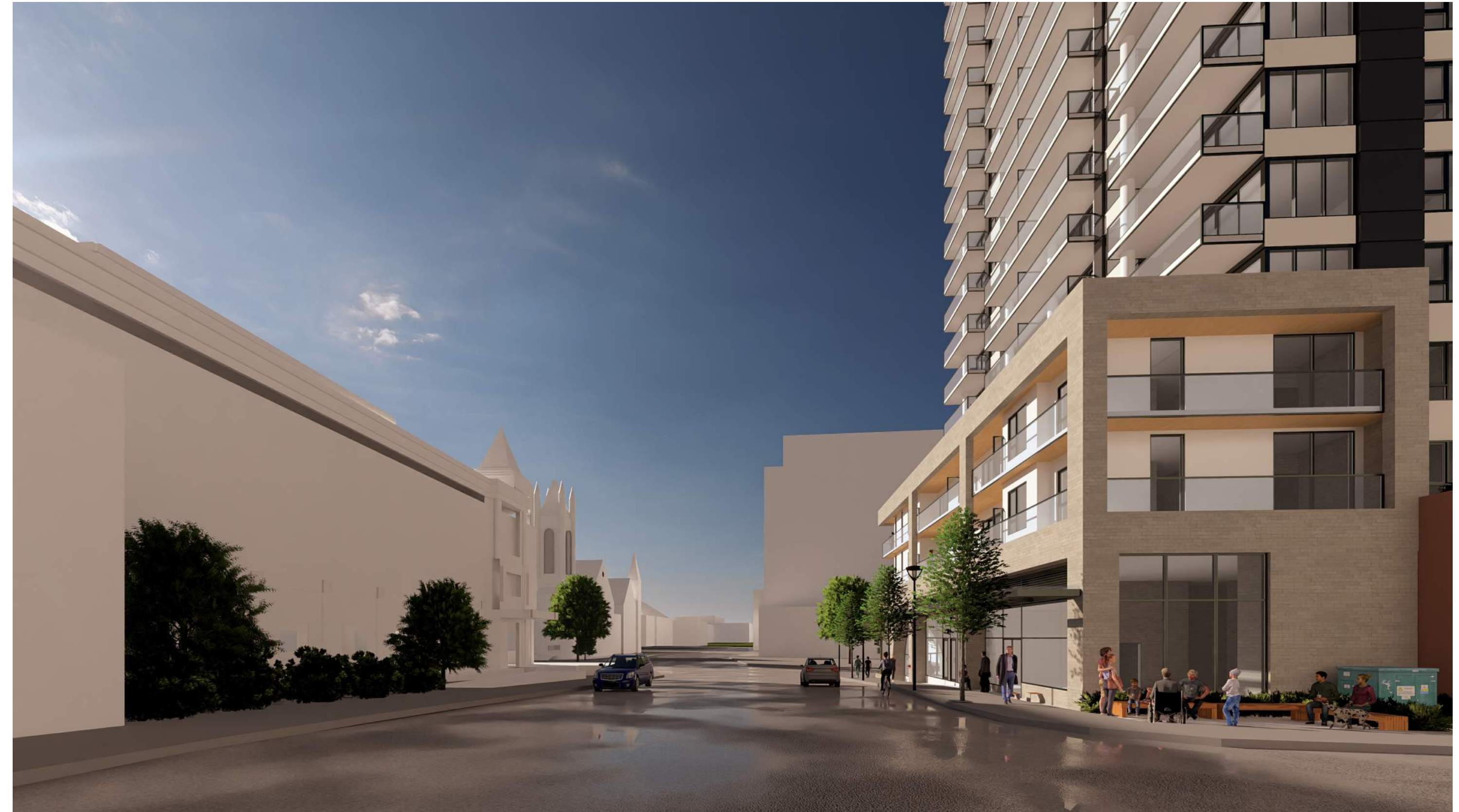
VIEW LOOKING SOUTH DOWN QUADRA ST
