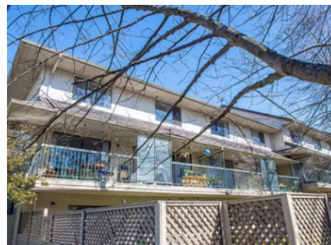
Current 38-unit townhouse complex.
