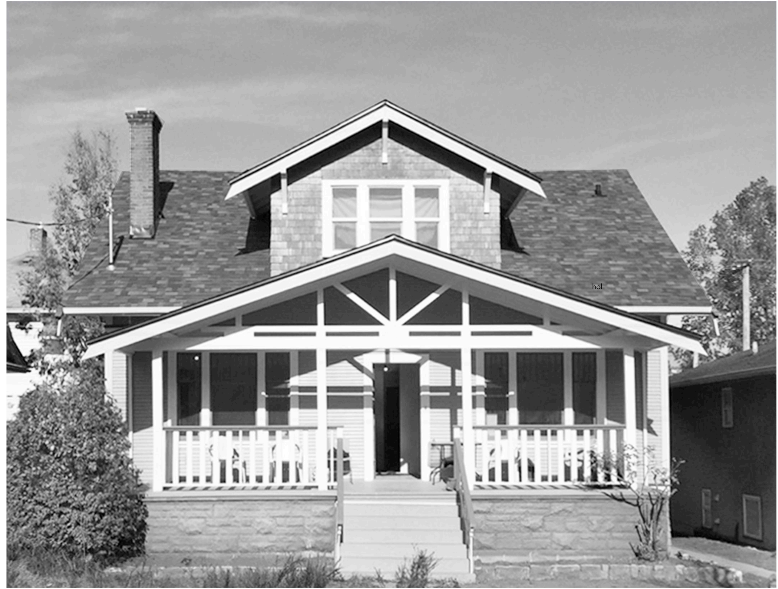
01 SOUTH ELEVATION PHOTO - EXISTING None
