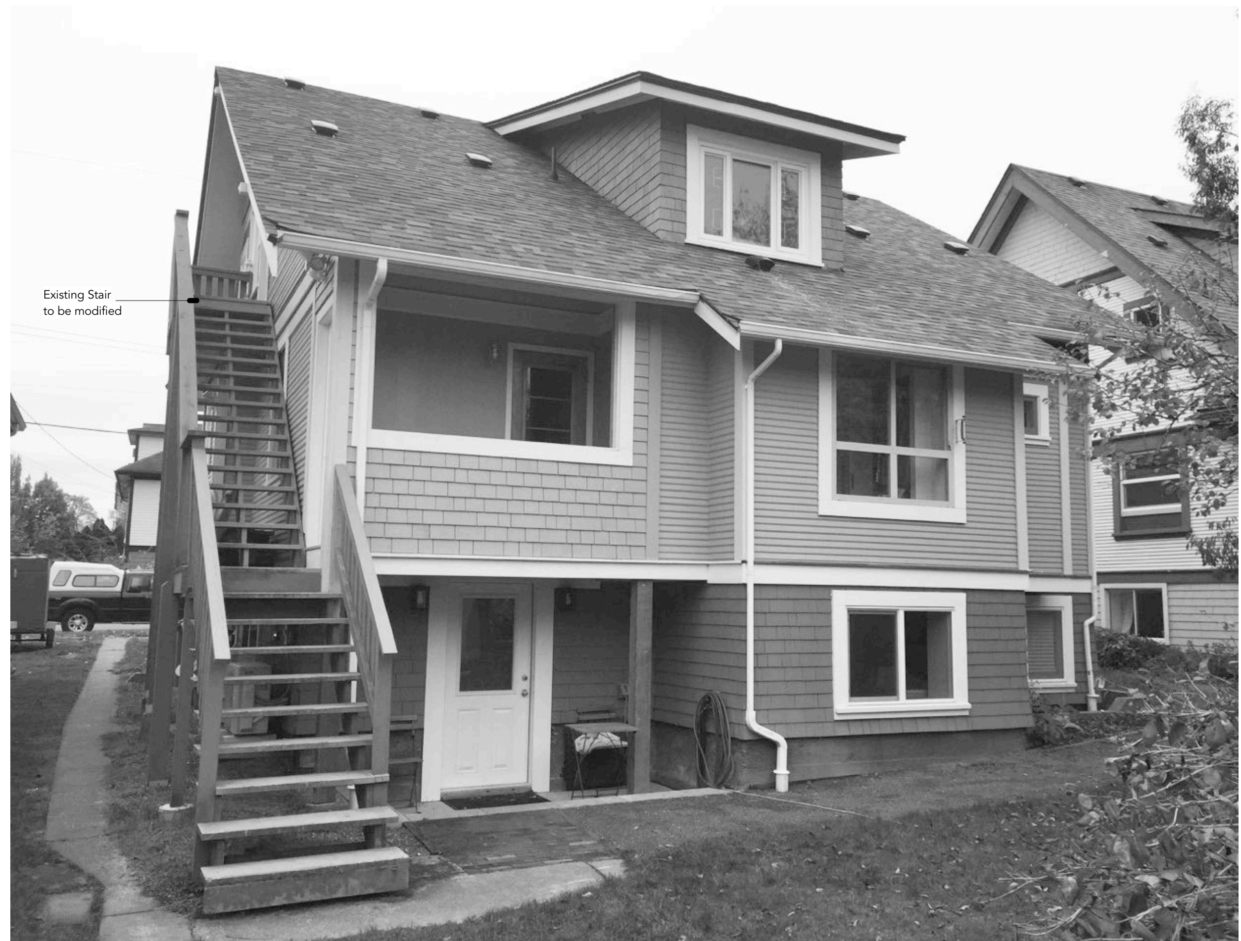
02 NORTH ELEVATION PHOTO- EXISTING None
