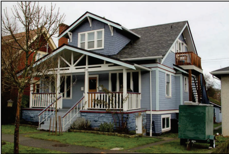
Front Elevation Facing Empress Ave (south)
