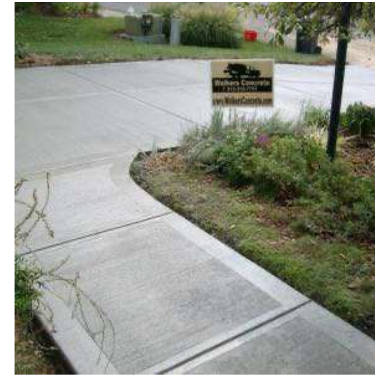
CIP CONCRETE PAVING
