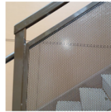
HANDRAIL & GUARD WITH PERFORATED METAL PANEL
