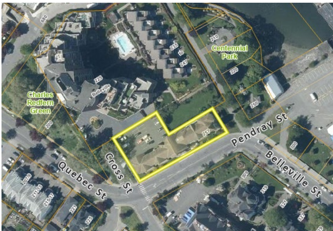
Figure 1: Aerial view of the subject site
