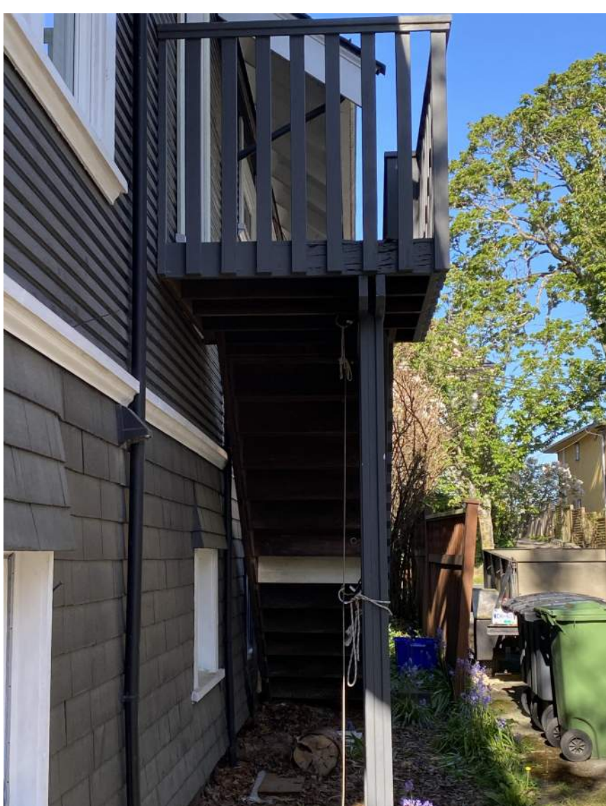
PHOTO 2: SIDE YARD STAIRS - EAST
