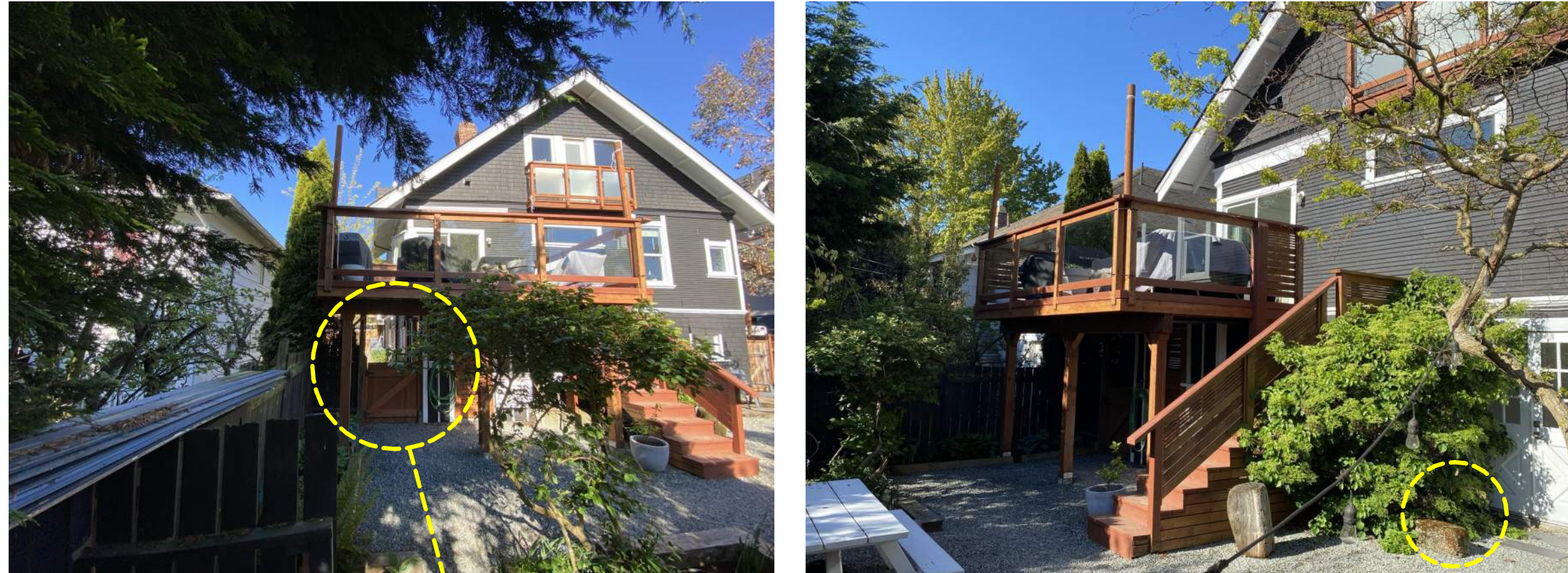
PHOTO 3: REAR DECK - EAST REAR/SIDE YARD ACCESS PHOTO 4: REAR DECK - NORTH EAST FOUNDATION OF DEMOLISHED ROOF DECK
