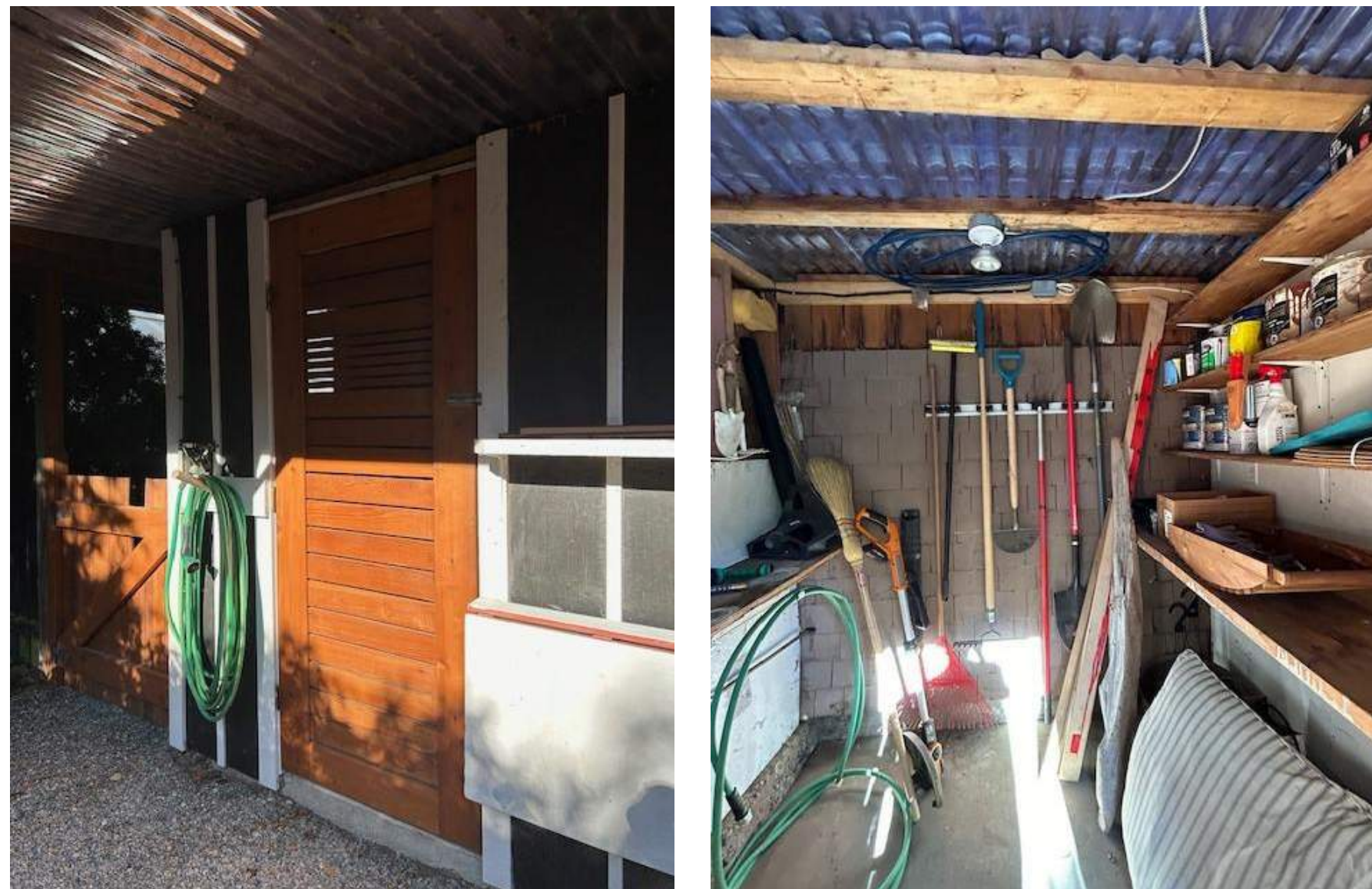
PHOTO 1: UNCONDITIONED SHED PHOTO 2: UNCONDITIONED SHED
