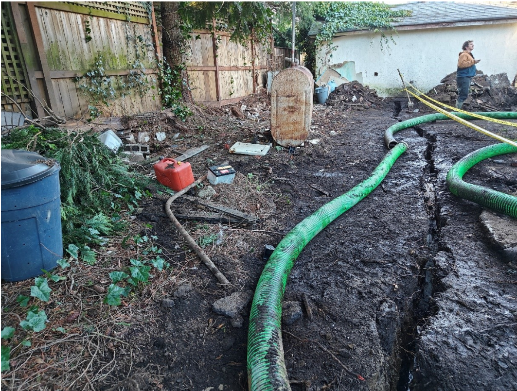
Figure 6 - Completed trench viewed from the northeast side of the property.
