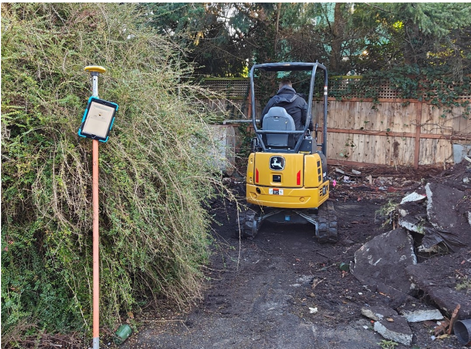
Figure 3 – Slab and building debris removal (January 15 th , 2025)
