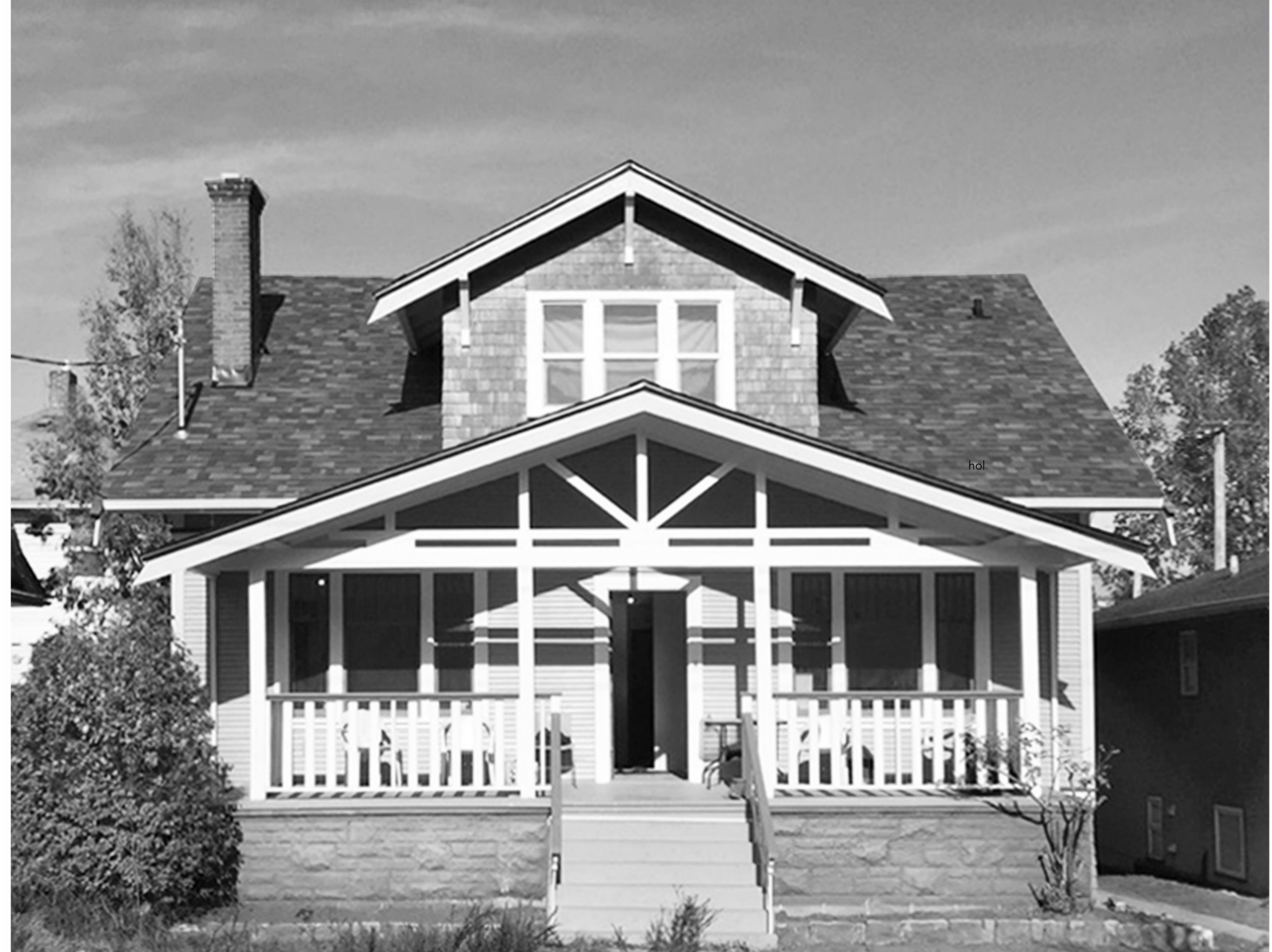
01 SOUTH ELEVATION PHOTO - EXISTING None
