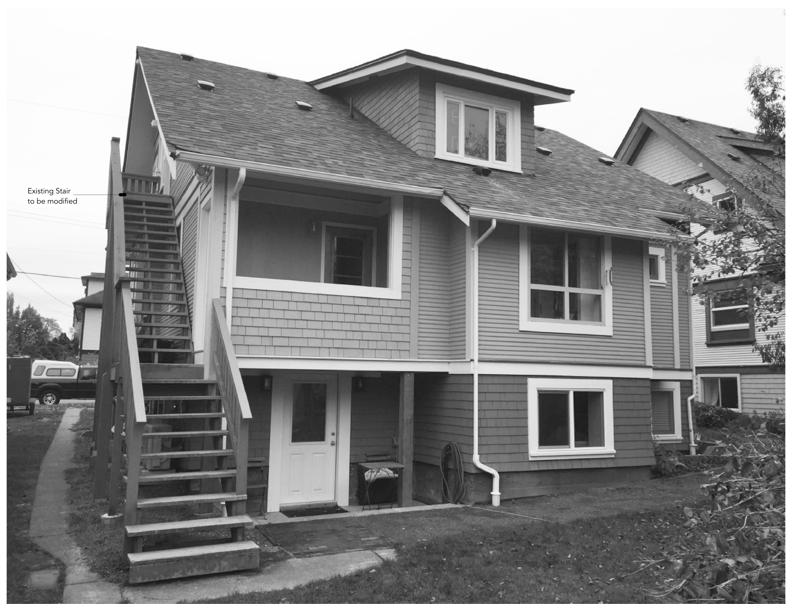
02 NORTH ELEVATION PHOTO- EXISTING None
