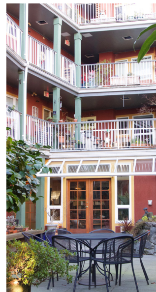
A single-loaded corridor configuration improves the livability of the inside corners on the L-shaped residential floors of this multi-family residential mixed-use building (left) and skylights and roof monitors enable these dual-aspect townhomes that are otherwise flanking a central community atrium (right.)
