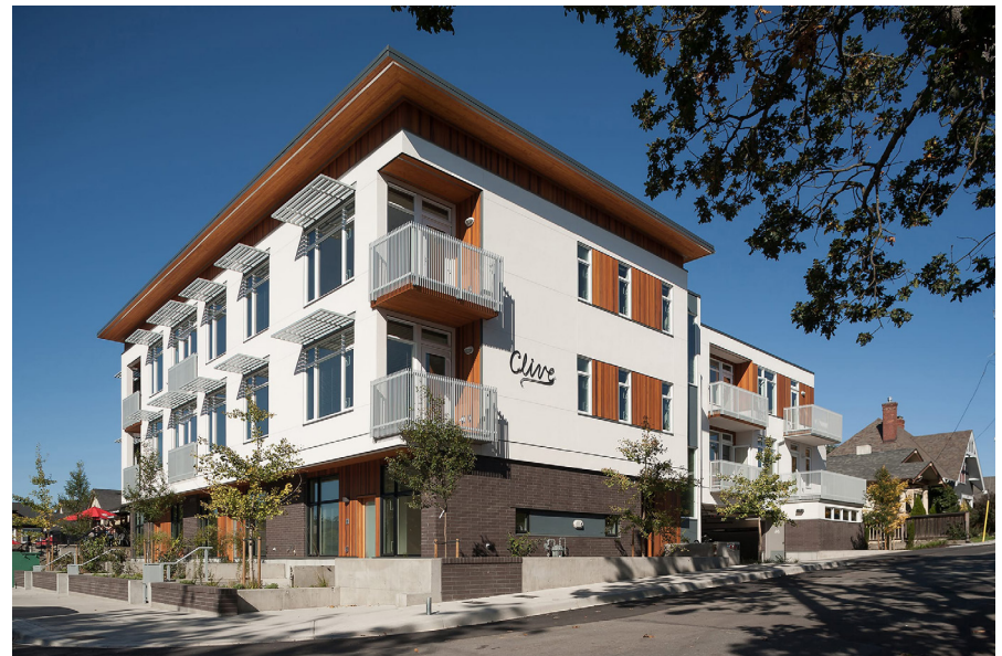
Different environmental control strategies for different elevations and solar exposures help improve building energy performance and provide occupant comfort at a multi-family residential development.
