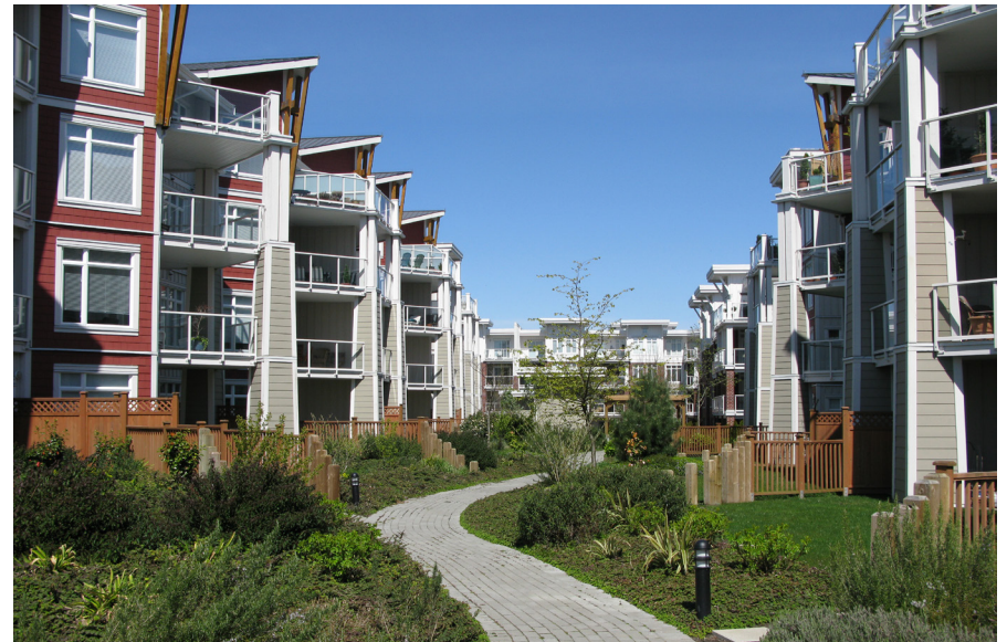
Built and conceptual examples show through-block walkways dimensioned and equipped to suit surrounding uses, building heights, natural features and vehicular access needs.
