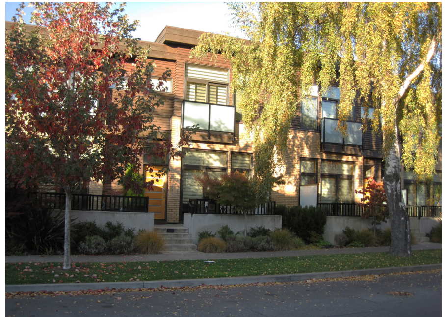
Reduced setbacks on a street with mature trees and a landscaped buffer.
