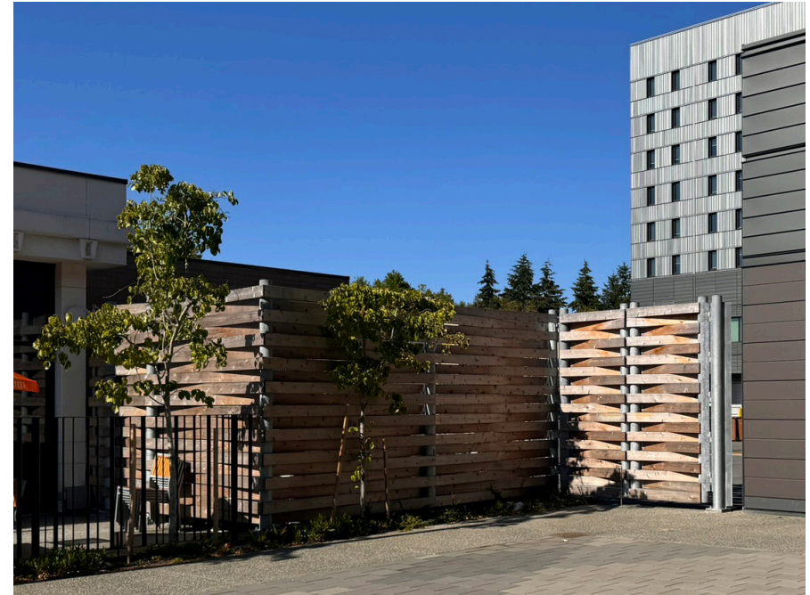
Screening at the public realm interface of a loading court serving multiple back-of-house areas of a mixed-use institutional-residential development.
