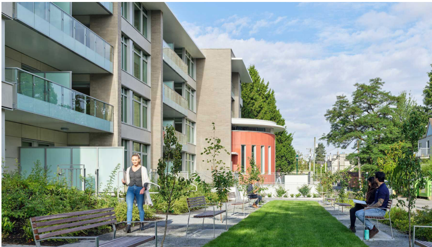
The top-floor step-back at a five-storey multi-family residential development helps improve solar access for the rear yard outdoor amenity area.
