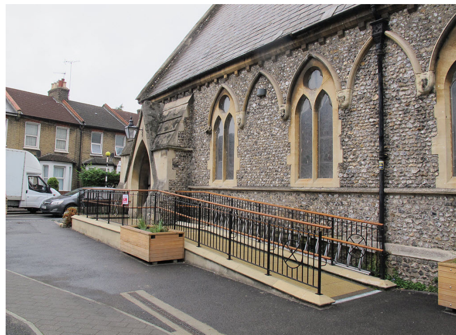
Access ramp and its elements are designed to be integrated into the building and site at a heritage church.
