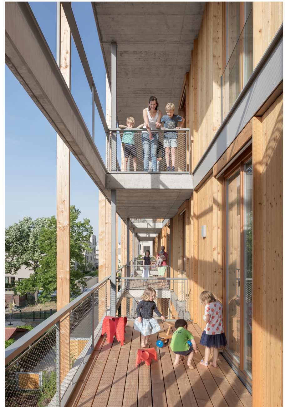
Thermally broken balconies and decks help create private and semi-private outdoor spaces for residents at a high-performance multi-family residential development.
