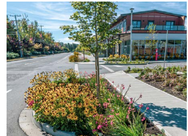
Boulevard rain garden Marigold Lands, Victoria BC
