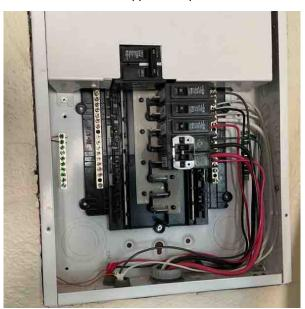
7.6.3 Branch circuits appear compatible with disconnect ratings. (unit 1)
