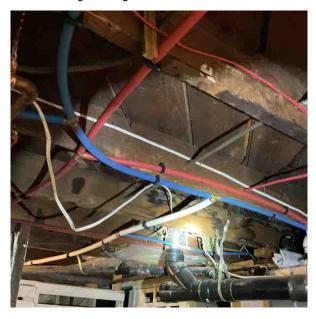
6.5.2 Stains throughout are evidence of past leakage. The stains are dry.
