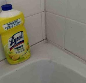
9.9.2 We detected excess dampness behind the wall finish indicating possible trapped moisture. This condition may cause concealed damage. Conduct further review as required, budget accordingly for repairs.
