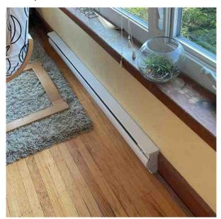
8.2.2 Heater did not respond to normal operating controls and appears to blow the breaker. Conduct further review. (unit 5)
