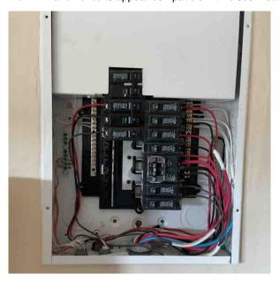
7.6.2 Branch circuits appear compatible with disconnect ratings. (Unit 3)
