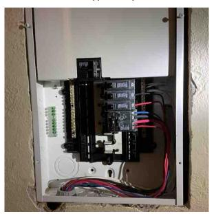
7.6.5 Branch circuits appear compatible with disconnect ratings. (unit 5)
