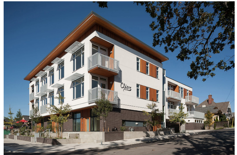
Different environmental control strategies for different elevations and solar exposures help improve building energy performance and provide occupant comfort at a multi-family residential development.
