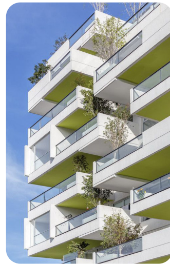
Examples of balconies located and designed to provide shade in summer and sunlight access in winter.
