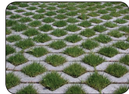
Image 17: 'Permeable Surface Design' Cellular Concrete Pavers in which natural grass can be grown
