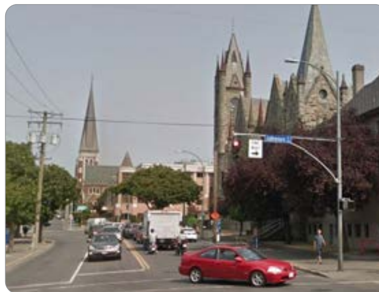
St. John the Divine Anglican Church in the background provides a terminated vista and landmark feature along Quadra Street.
