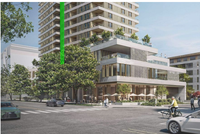
Figure 4: Location of vertical break in west façade (shown in green)
