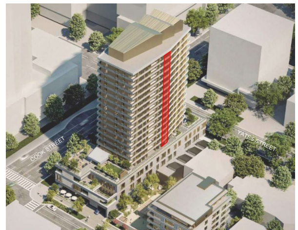
Figure 5: Suggested location of vertical break in west façade (shown in red)
