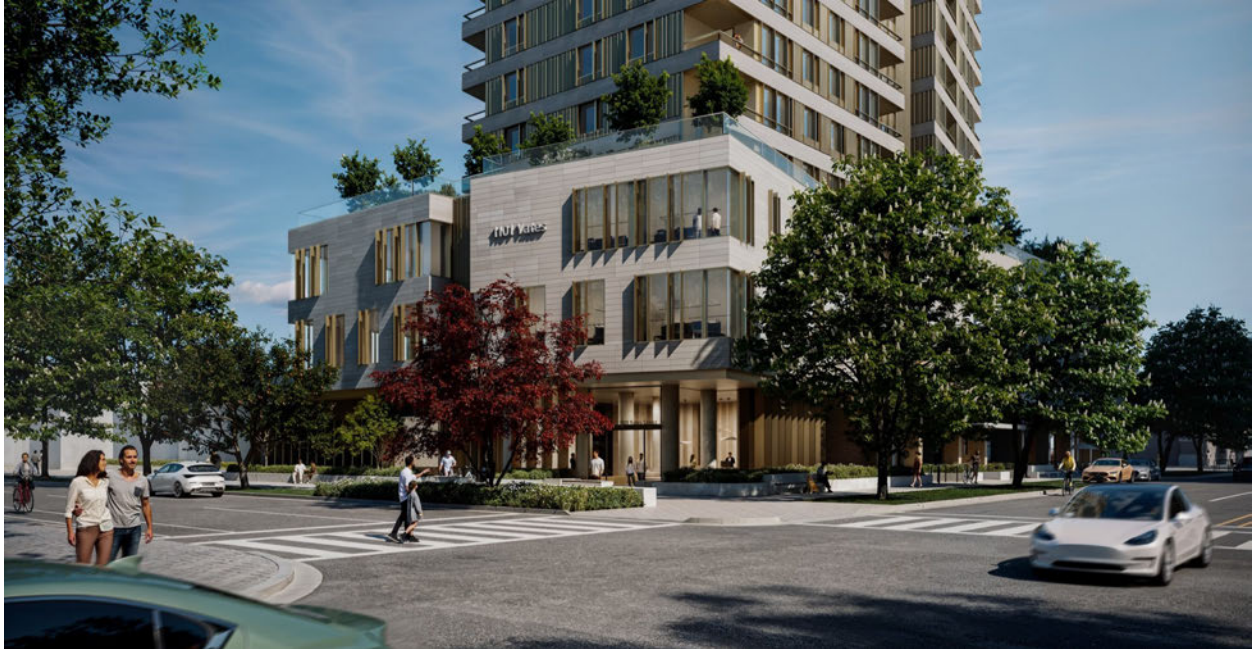
The commercial office entrance defines the landscaped plaza at the corner of Yates and Cook Streets.
