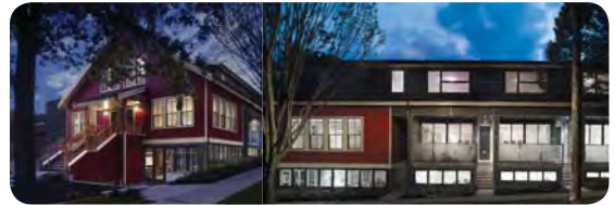
In this example a heritage school house was converted into townhouses. Photos show the front (left) and side (right). The school house was lifted to allow for additional units below.
