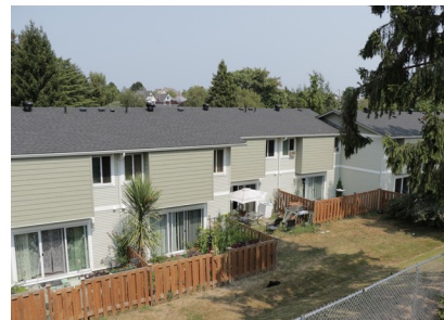
Two larger housing cooperatives – Tyee and Pioneer – add to the diversity of housing options.
