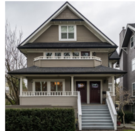
Figure 27: Example of heritage house converted to a duplex
