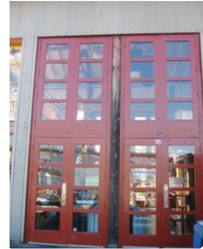
Figure 34. Example of light industrial frontage which creates an interesting and pedestrian friendly environment (see policy 7.3.1).
